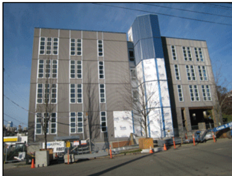
Comfortable urban lofts for artists under construction in Seattle
